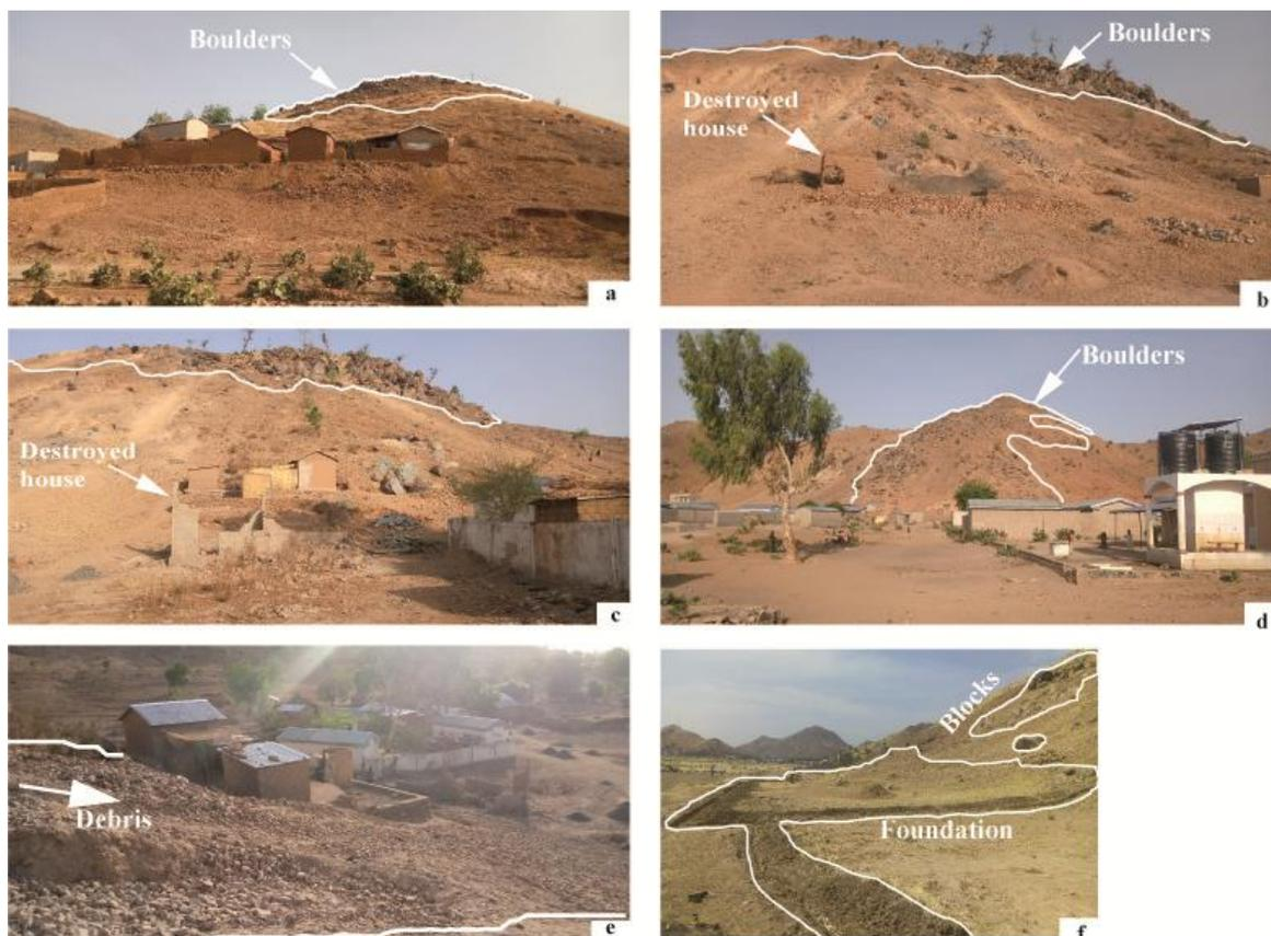
**Figure 6:** Pictures of different vulnerability in DV: **a, b, c** and **d**) houses exposed to rock fall; **e**) houses exposed to debris falls; **f**) foundations exposed to the rock fall.
